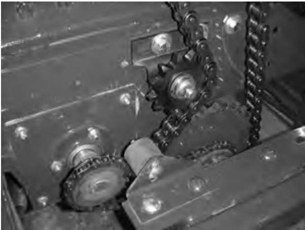
Figure 41 - Mill To Mixer Auger Drive Chain.
